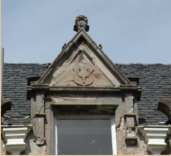
Fig. 1-2.: One of the pediments: pediment with shield and stags head. Before and after conservation. (Stones cut by the stone mason)
