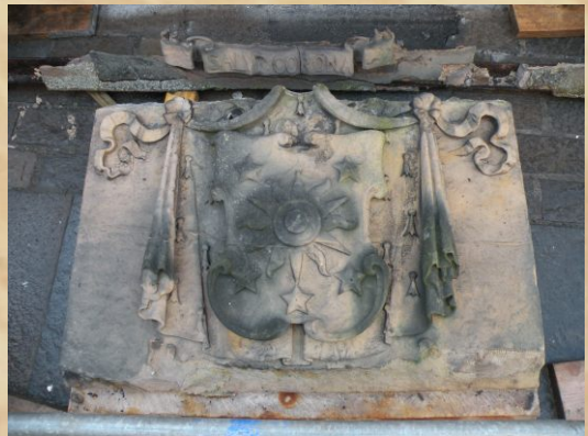
Fig. 76-77.: Dingwall Town Hall Balcony. Conservation of the main part. Report with recommendations how to proceed with each stone, Steam cleaning, removal of old resin repairs, consolidation of delaminations, acrylic mortar and lithomix repairs, inserting stainless steel armatures into delaminating stones.
