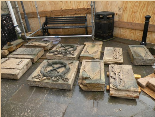
Fig. 76-77.: Dingwall Town Hall Balcony. Conservation of the main part. Report with recommendations how to proceed with each stone, Steam cleaning, removal of old resin repairs, consolidation of delaminations, acrylic mortar and lithomix repairs, inserting stainless steel armatures into delaminating stones.
