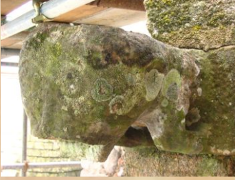
Fig.: 14-15.: Gargoyle before and after cleaning and conservation. Chin of the gargoyle was re-attached.
