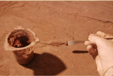
Fig. 60-63.: Conservation of XIV century Tombgrave including: steam cleaning, desalination, consolidation of delaminations using solutions of Paraloid B72 mixed with acetone and IMS (methanol), acrylic mortar repairs, Base making to provide firm and even support for the stone.
