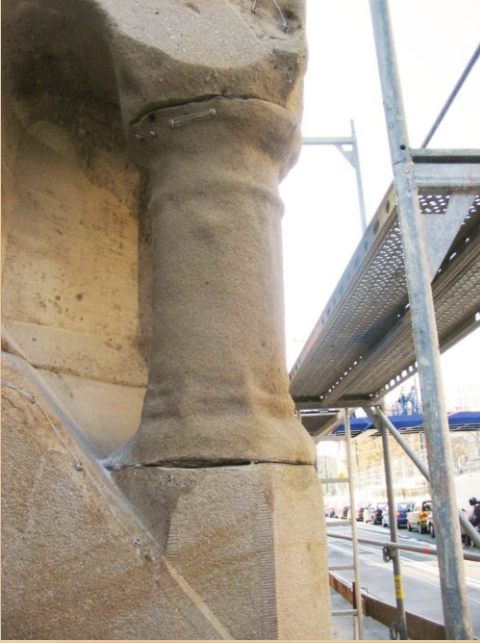
Fig.: 26, 27.: Cracow; Reconstructions made using stainless steel armatures and two ready made mixes by Baunit and Remmers, upper part mixed with Remmers Hafffest for better adhesion.
