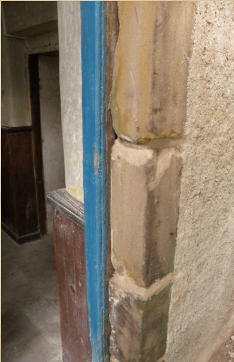
Fig. 64-67.: Lime mortar repairs on window and door surrounds.
